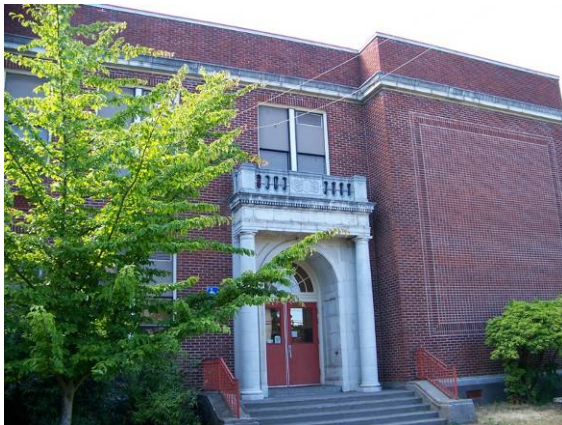
North side of east (front) elevation, looking west.
