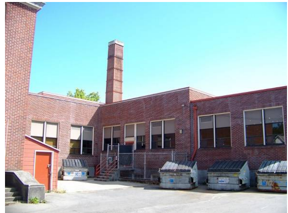
West (rear) elevation at cafeteria, looking southeast.
