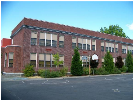
South (side) and west (rear) elevations, looking northeast.
