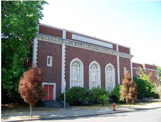
East (front) elevation, looking west.
